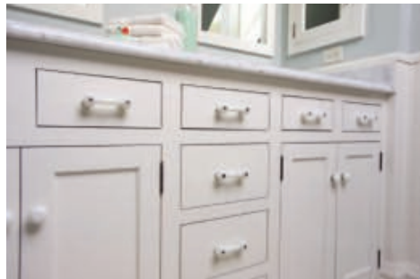
Old and new knobs. Can you tell which of these pull handles are 80 years old and which are reproduced? The couple ordered reproductions through salvage stores and on the Internet. The new pull handles are the two on the far-right drawers.
